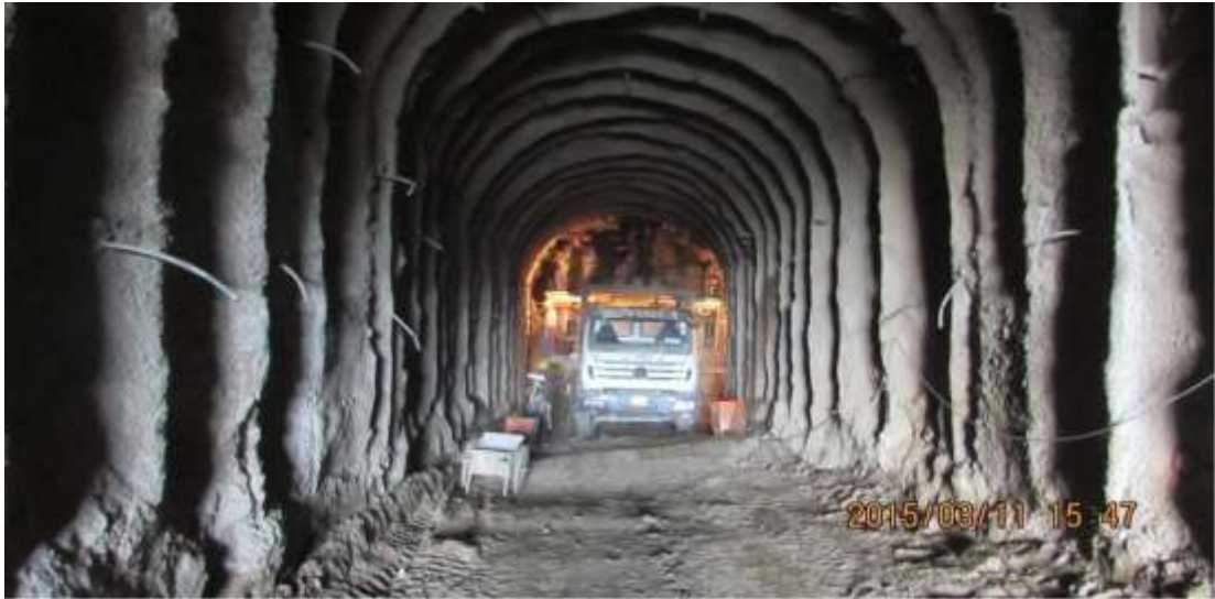
Adit 6 Excavation works
