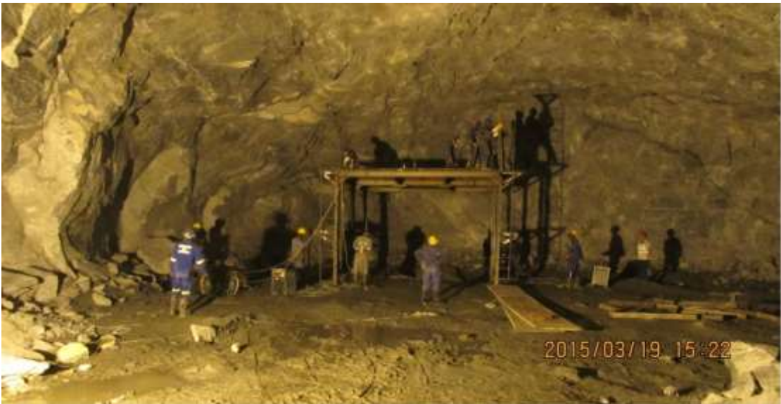
Power House Excavations
