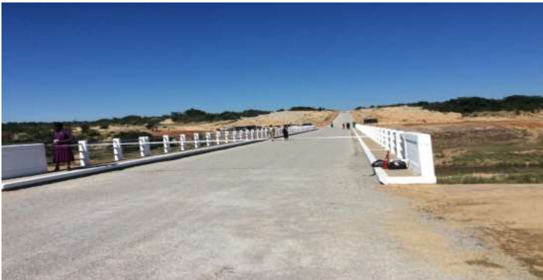
Save Bridge and Roadworks which were commissioned by Vice President Phekezela Mphoko on 25 March 2015
