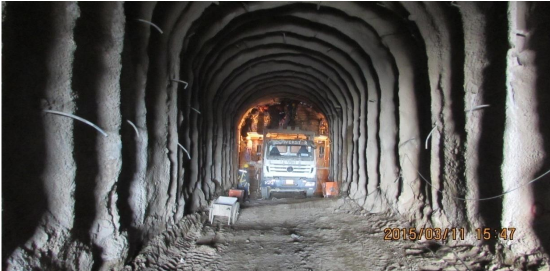
Adit 6 Excavation works
