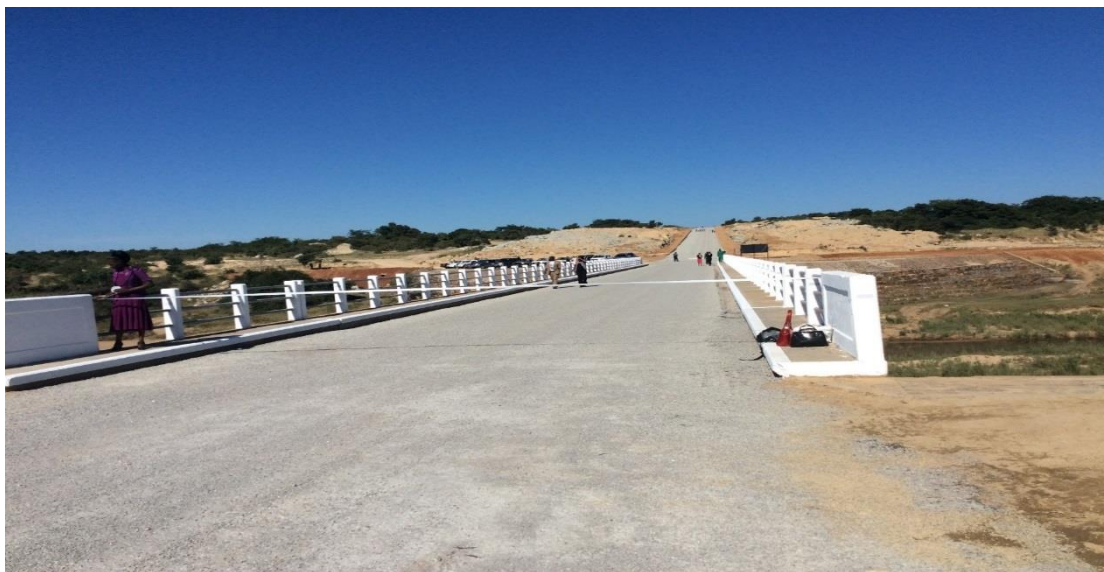
Save Bridge and Roadworks which were commissioned by Vice President Phekezela Mphoko on 25 March 2015
