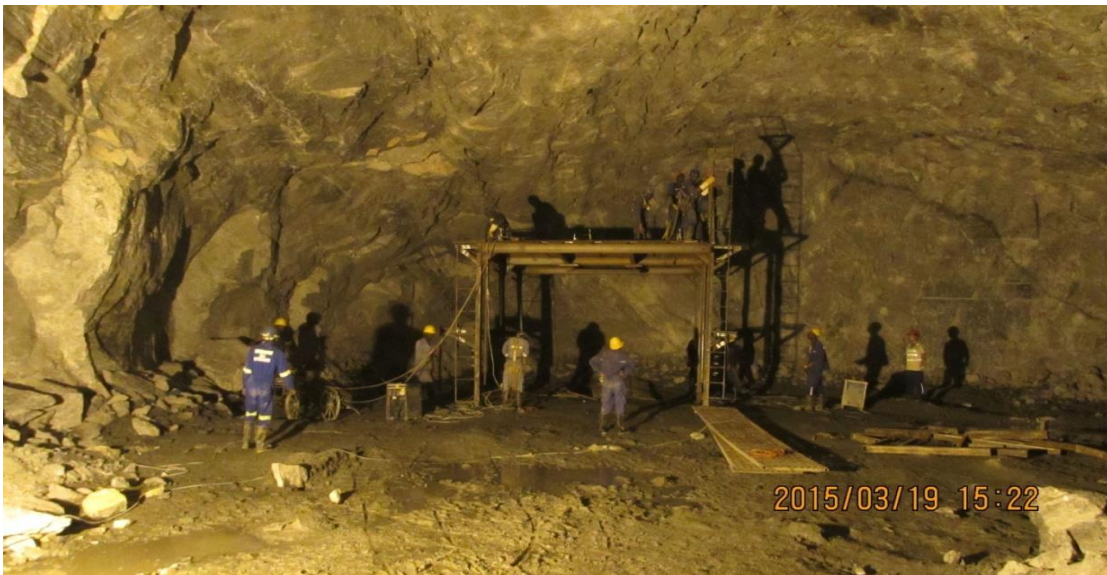
Power House Excavations
